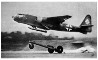
a skid proved to be a bad idea and required a major re-design to correct. Once the problems were sorted out the AR-234 got into production in early 1944 as the world's first operational jet bomber.
